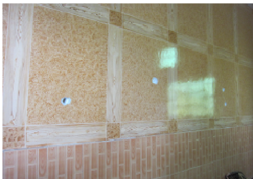
Bullet holes in the wall at about head level are visible in the room where the bodies of Mohamed 'Awad 'Abd al-Qader, Ahmad Ja'afar and Iyad Ghneim were found, their hands still tied at the back with plastic cuffs. ©Amnesty International
